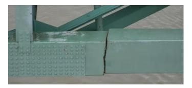
On May 11, a contractor for the Arkansas Department of Transportation discovered a crack in a steel support beam while inspecting the <u>Hernando de Soto Bridge</u> (pictured above), a 48-year-old span on Interstate 40 that crosses the Mississippi River, connecting Arkansas to Tennessee.
