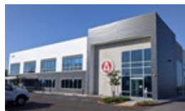
AGC East County Facility & Apprenticeship Training Center
